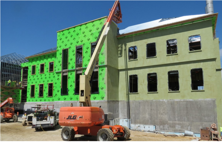
Vapor barrier installation with spray or roll-on.
