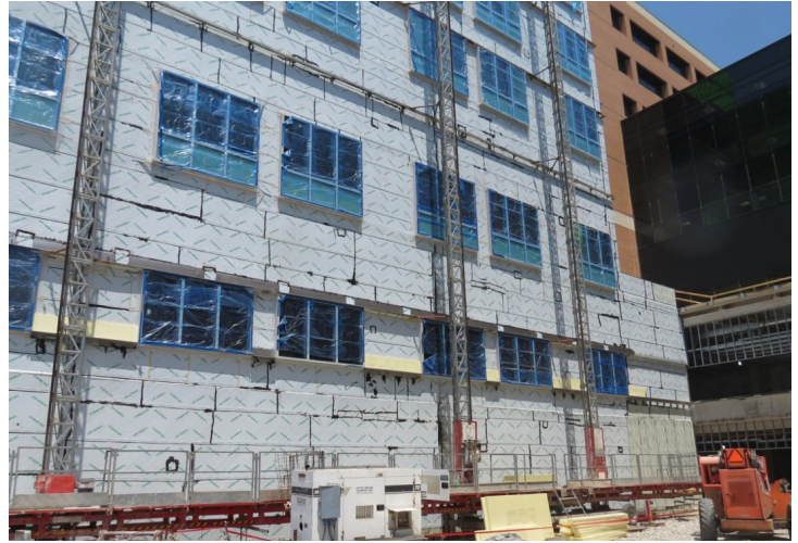
Vapor barrier installation with self-adhered sheets.
