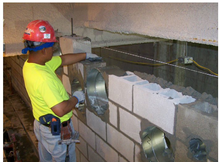
A bricklayer installs mechanical duct sleeves at precise locations per the BIM model as he construction the masonry.
