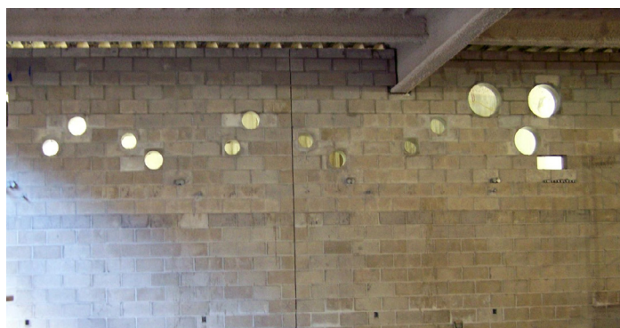
As the concrete masonry was constructed, the bricklayers installed 468 sleeves for HVAC, 69 sleeves for electrical, 159 sleeves for mechanical pipe, 257 sleeves for fire protection, 231 sleeves for plumbing, 343 sleeves for water, and 10 sleeves for miscellaneous, resulting in a total of 1,537 sleeves in the masonry walls.
