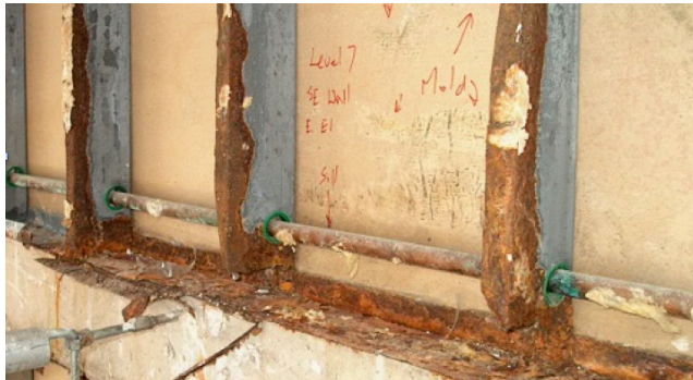
Corroded steel studs and tracks within the exterior wall of a multi-family building undergoing a full enclosure rehabilitation in Climate Zone 4 as a result of water ingress into a wall assembly with low drying potential.
