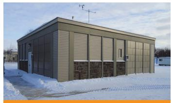
**Wall Assembly Research Center:** A laboratory built by The Dow Chemical Company in Midland, Michigan to test the performance of several different wall assemblies in real world conditions.
