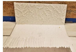
To verify proper coverage and embedment, lift a tile and examine the back of the tile for mortar coverage, and examine the substrate for ridge collapse. This photo is an example of ideal coverage and embedment.
