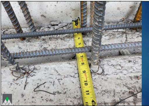
Rebar Coverage and Allowable Tolerance
