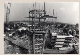
curved steel columns and 13 horizontal loops. The columns are joined at the main shaft by a tension ring at the top of the sphere and a compression ring at the bottom. The structure has been transformed by several renovations but many of the features listed above can still be observed today.
