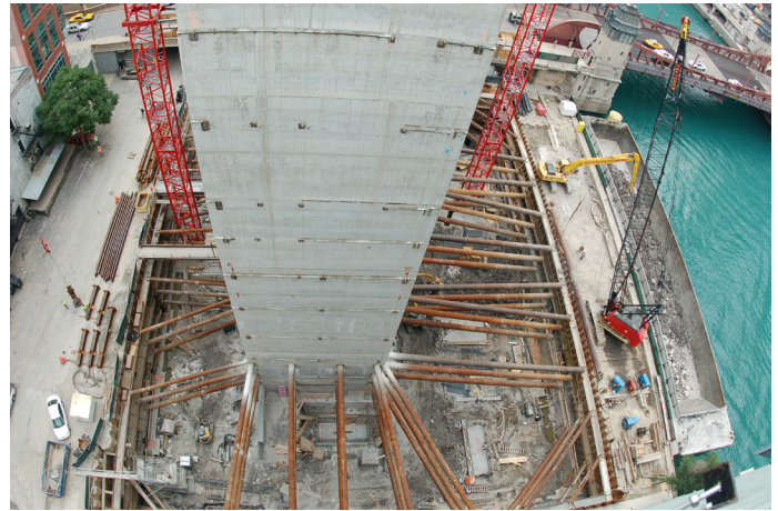
Photo of the earth retention system at 300 N. LaSalle provided by Thatcher Foundations, Inc.
